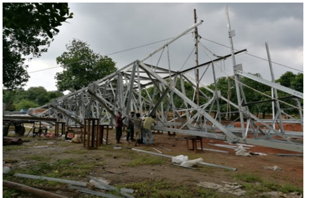
TOWER ASSEMBLY AT FACTORY PREMISES
