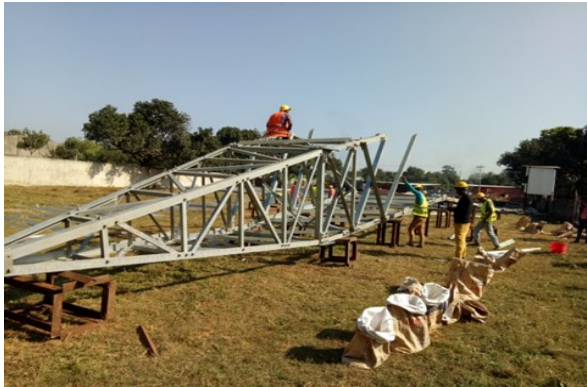
TOWER ASSEMBLY AT FACTORY PREMISES
