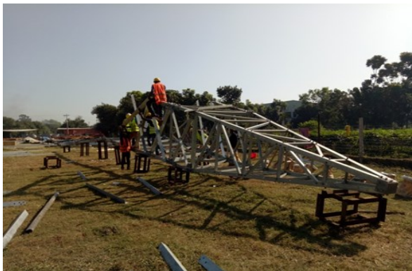
TOWER ASSEMBLY AT FACTORY PREMISES
