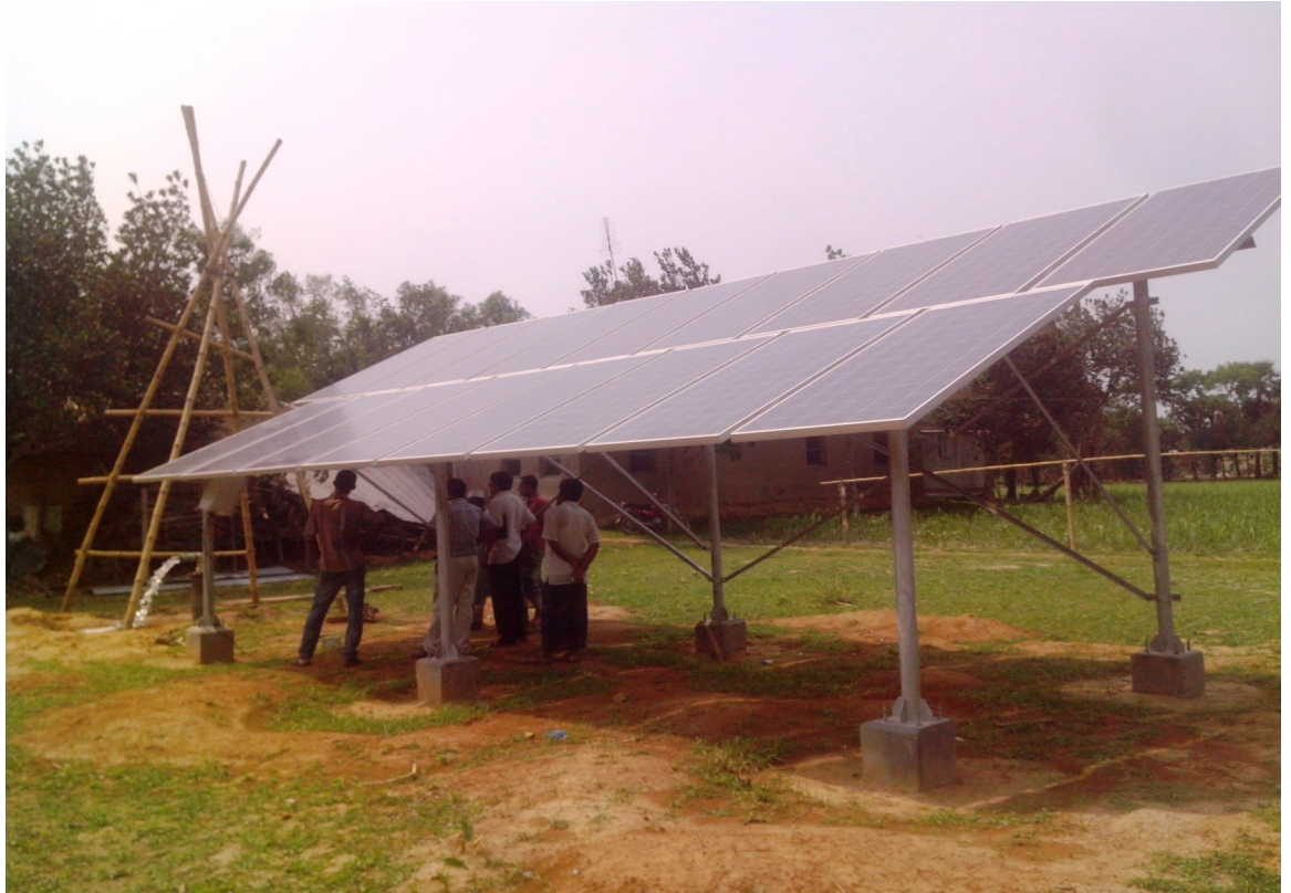
5KW Solar Power Pump with Mounting Frame Structure project for PUMP-1 at Lohadi, Kapashia, Gazipur.
