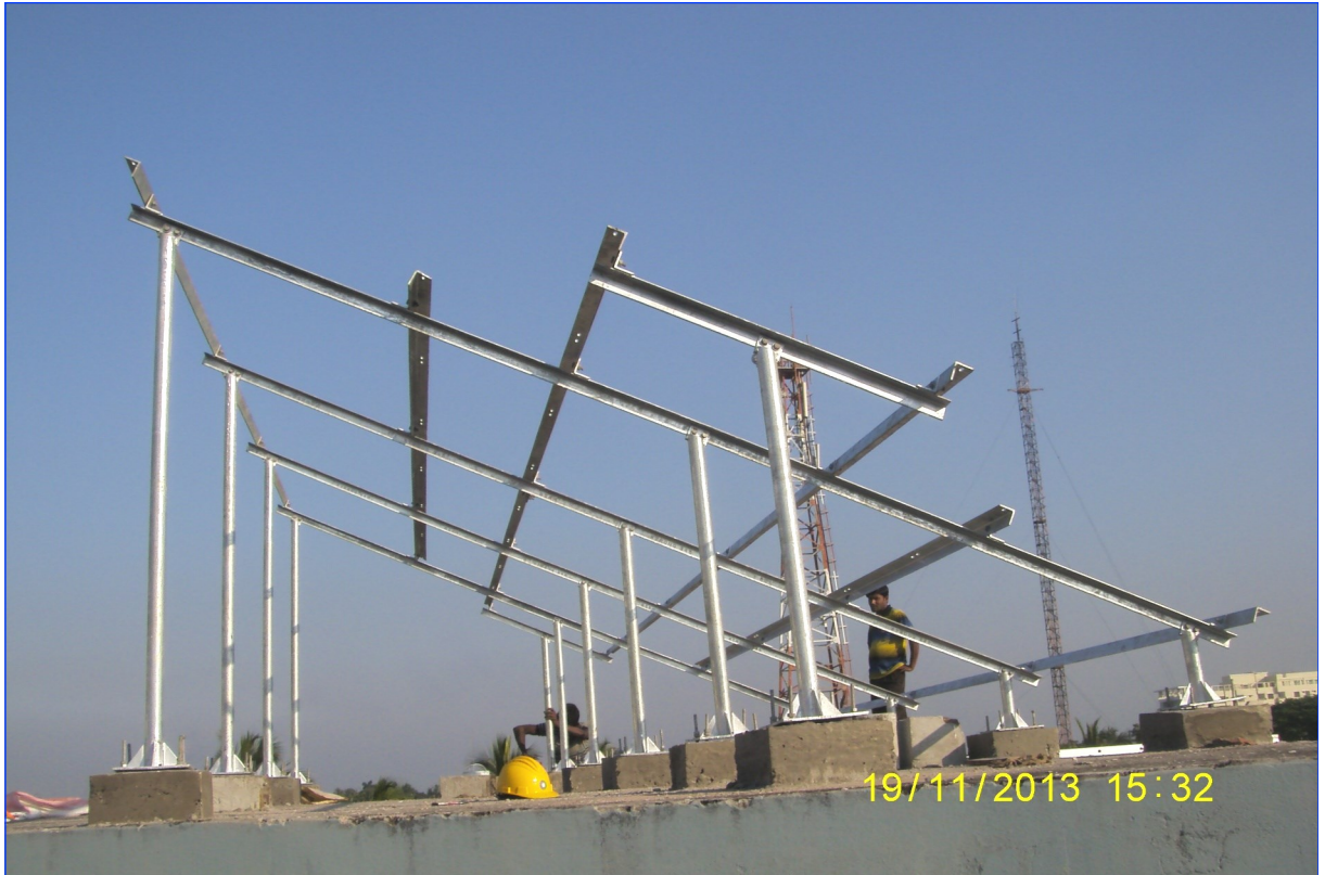
Solar Panel Mounting Frame Structure at Bangladesh Bank, Khulna Branch, Khulna (5 Kw Project)
