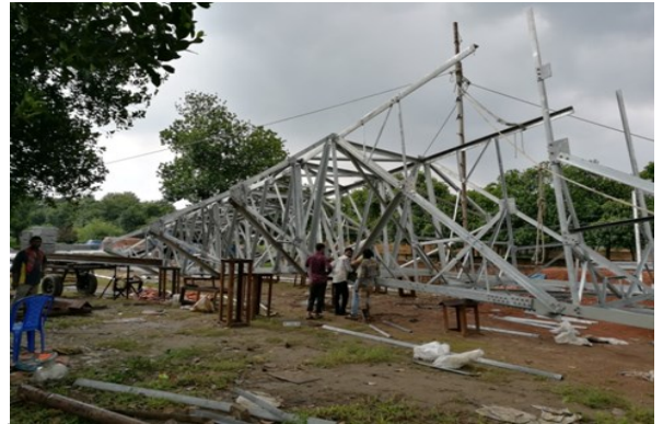
TOWER ASSEMBLY AT FACTORY PREMISES
