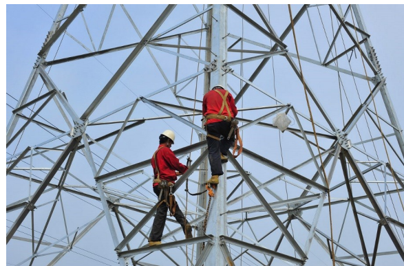
TOWER ASSEMBLY AT FACTORY PREMISES
