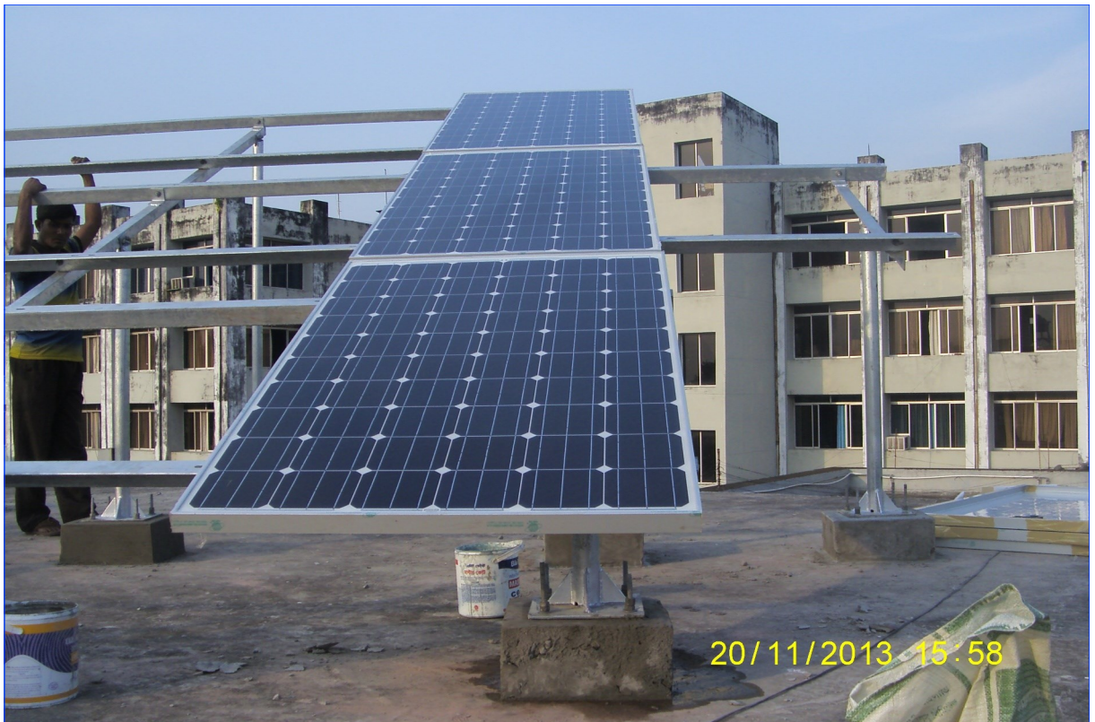
Solar Panel Mounting Frame Structure at Bangladesh Bank, Khulna Branch, Khulna (5 Kw Project)
