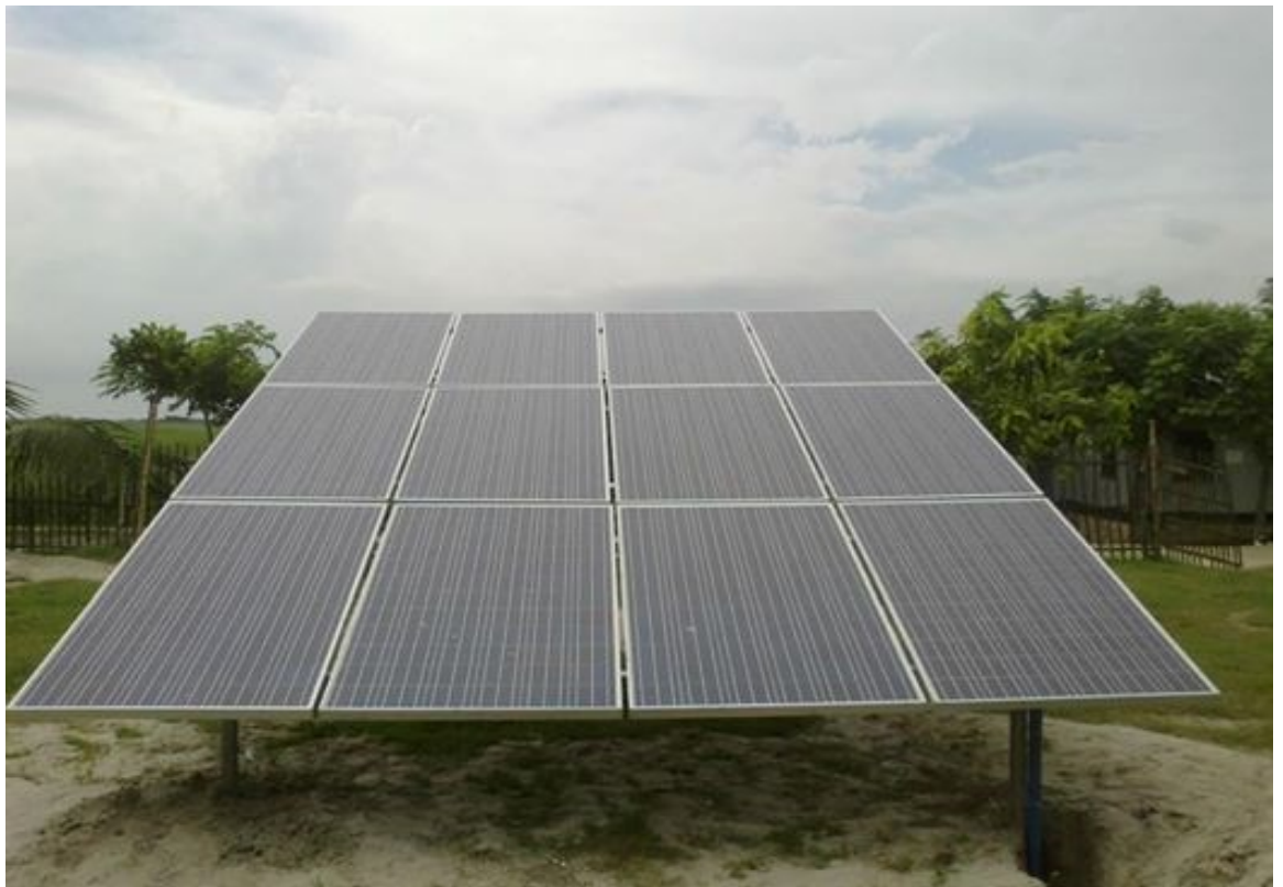
3KW NANO GRID Solar Power plant with Mounting Frame Structure project for K-4 at Vagjot Bazar, Daulotpur, Kustia.
